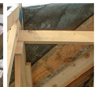
Mould damage because of trapped moisture
